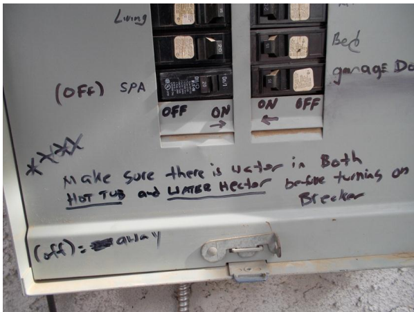
Figure 10. Before you begin to empty the hot tub, turn OFF the SPA breaker . Warning, if the hot tub is empty of water and the SPA breaker is on, you will damage the hot tub.
