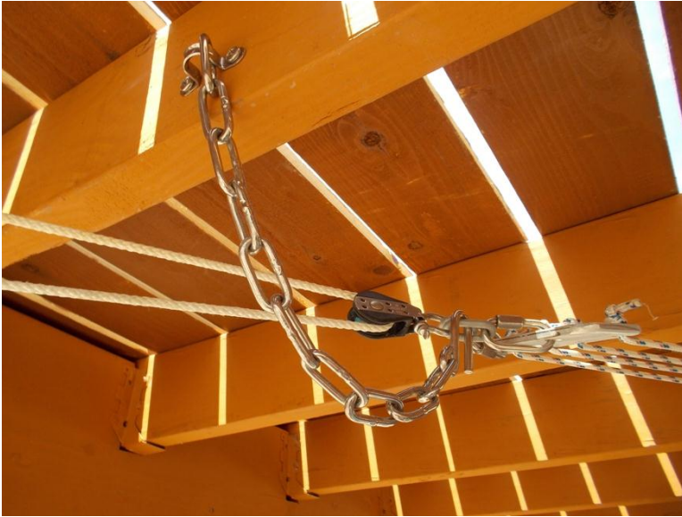
Figure 6. The crank has a clutch that keeps it in the up position automatically but just to be sure the cover doesn't accidentally fall when the hot tub is occupied, please place the chain tether on the pulley systems as shown in this figure.
