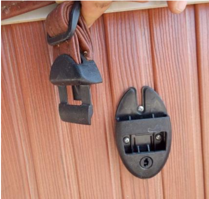
Figure 3. Snap buckles hold the cover on the hot tub, unsnap all these. I think there are at least four, please make sure you get them all.
