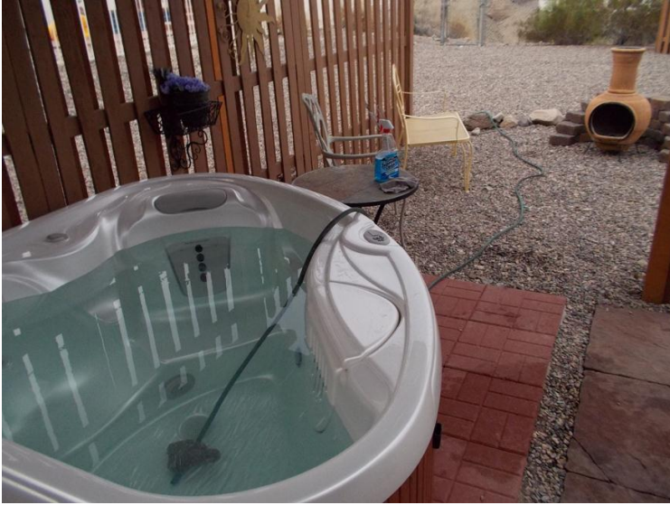
Figure 11. Siphon hose used to empty the hot tub. The end of the hose is out past the Chiminea (wood burner).
