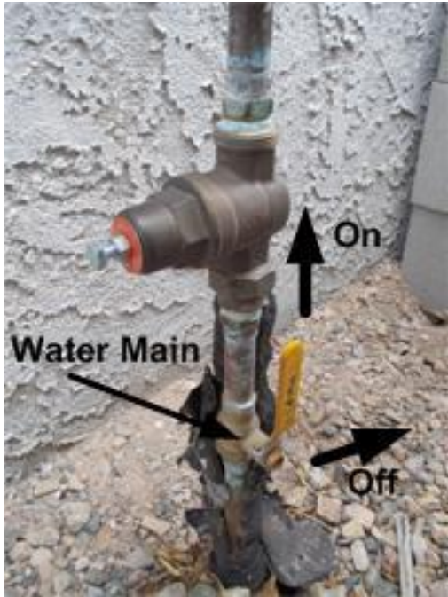
Figure 15. Turn OFF (horizontal position) the water main.
